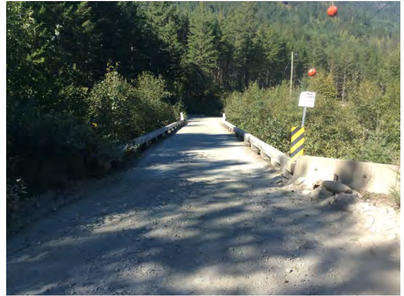
Approach from Right Bank when facing downstream
