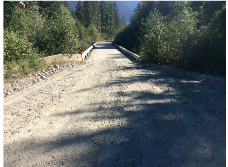
Right Bank Abutment when facing downstream
