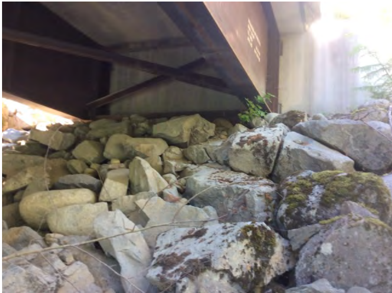
Left Bank Abutment when facing downstream
