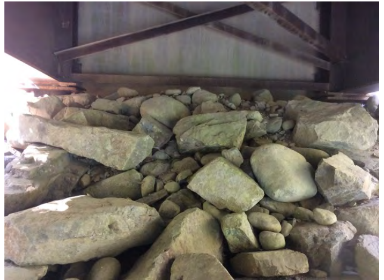
Left Bank Abutment when facing downstream
