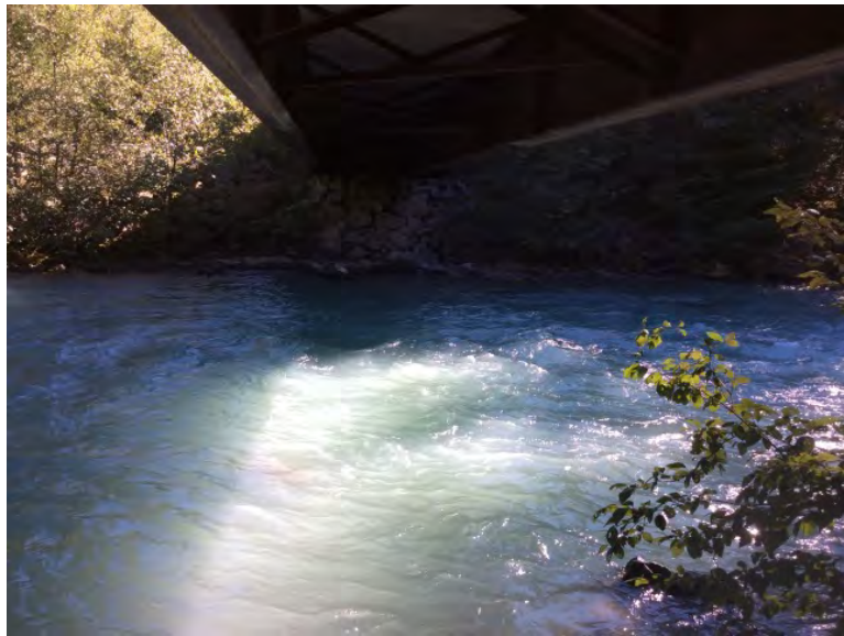
Right Bank Abutment when facing downstream
